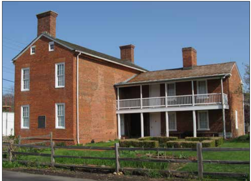
The Orange Johnson House of the Worthington Historical Society. A grant from the Ohio History Fund helped the Society replace the roof over the “porched” rear of the house, built in 1811. Photo courtesy the Worthington Historical Society. Unless noted, all images are from the Worthington Historical Society.
