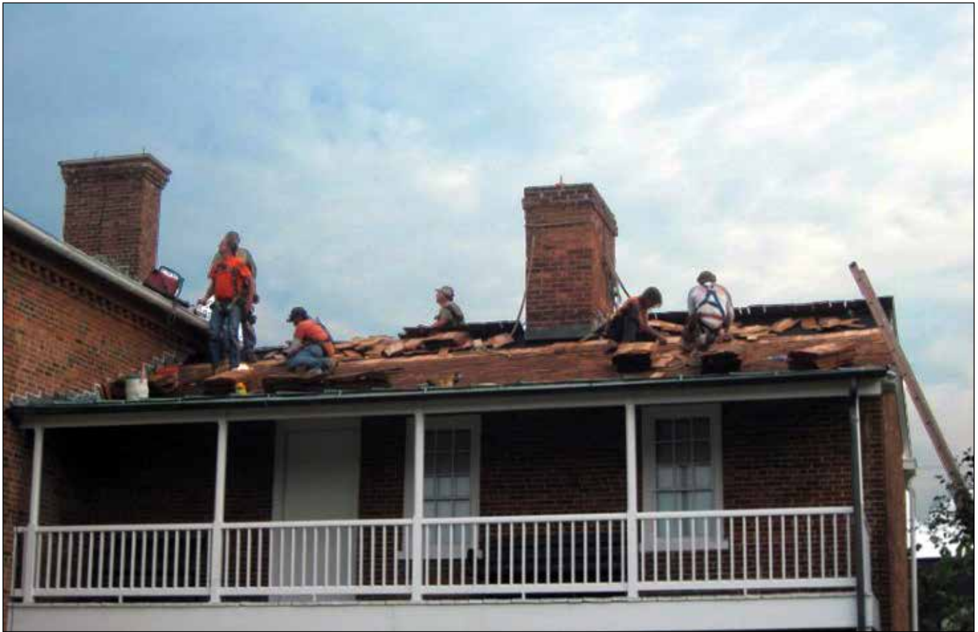
"During." Roofers proceeding with the work.
