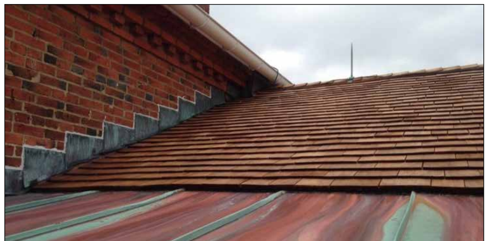
"After." A section of the new roof.
